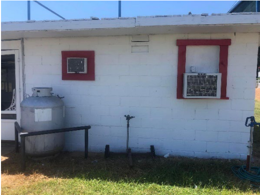
Remodel east concession continued
