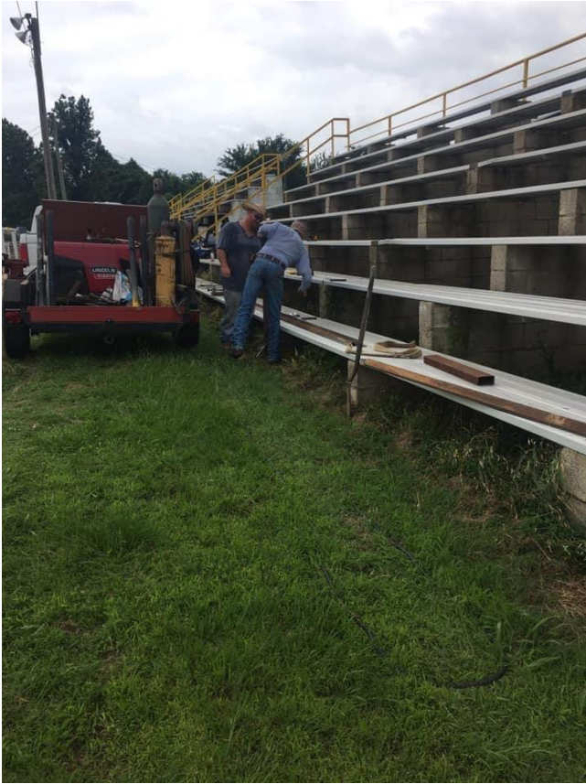
Installed safety hand railing on bleachers
