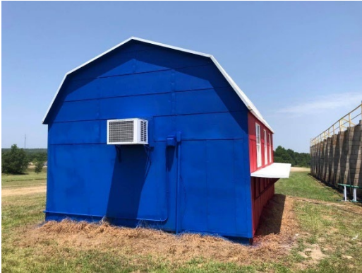
Fresh paint on west concession
